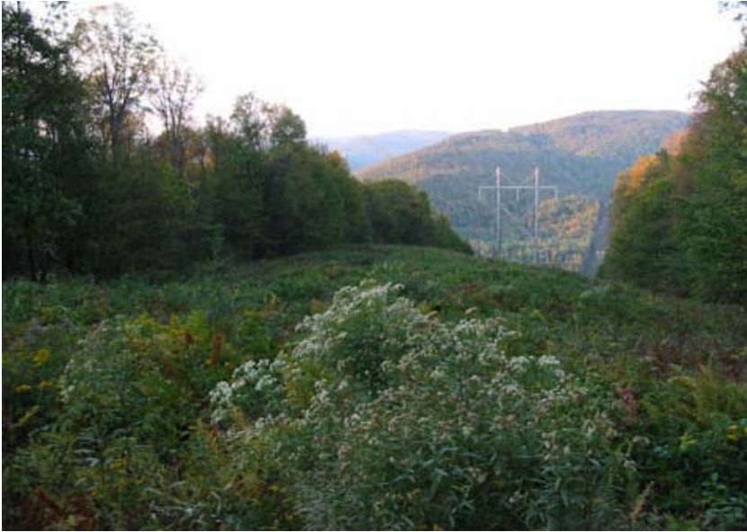
Stoddard Hill power line facing north
